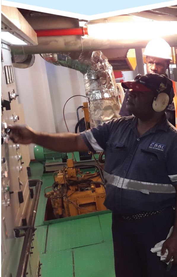
NMSA Ship Inspectors conducting ship inspection in the engine room.
