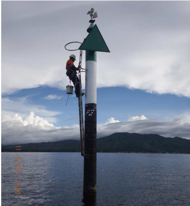
● AtoN Kimbe No.2 structure currently in place. Pile is a 600mm diameter
