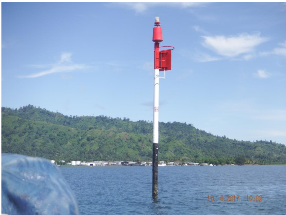
● AtoN Kimbe No.5 structure currently in place. The pile is a 180mm diameter.
